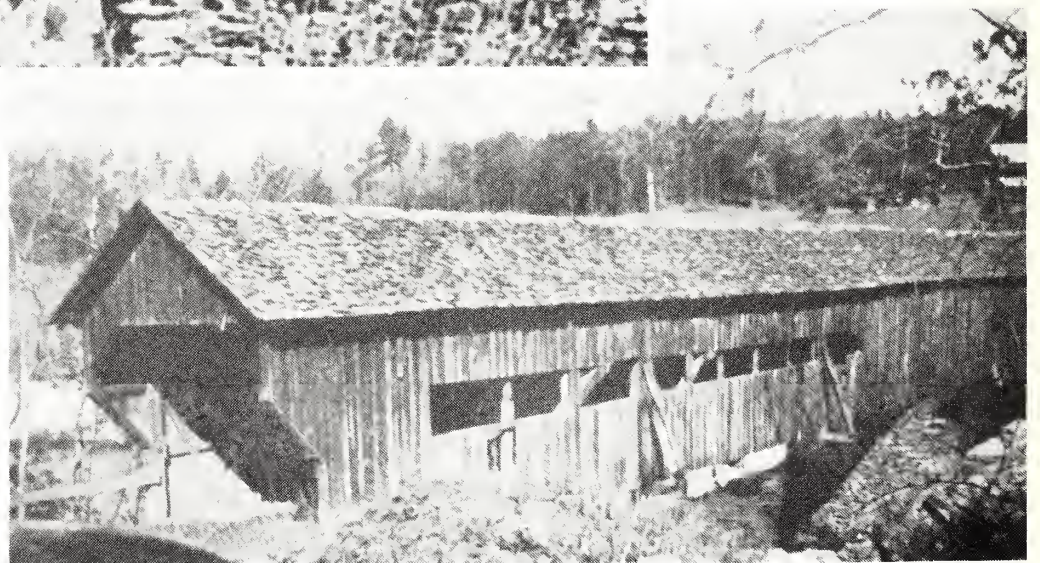
61) Covered Bridge @ Campbell Mill
